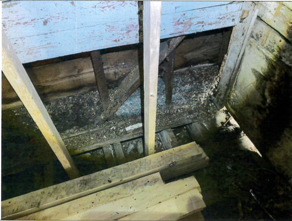
Photograph 3 – View of interior of south exterior wall. Note water staining at wall boards, stone between wall studs, and daylight visible at the southwest corner.
