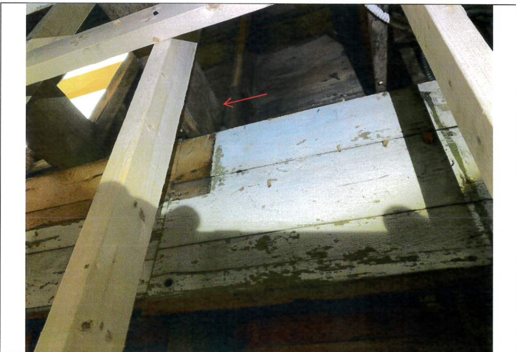
Photograph 12 – Close-up view second floor joists at south (front) exterior wall from below. Note not all second-floor wall studs were attached to the floor joists.
