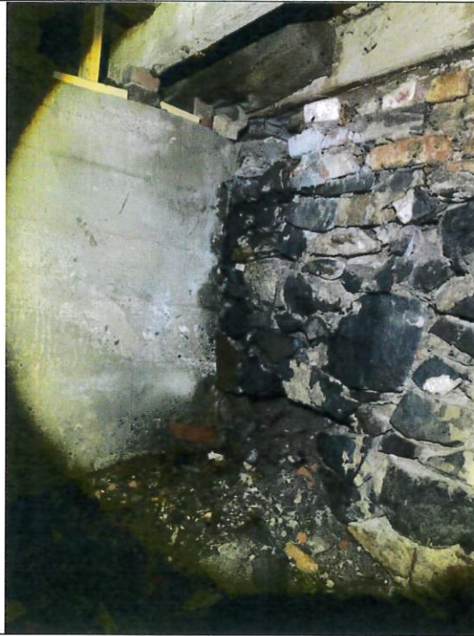
Photograph 21 – View of foundation at southwest corner. Note partially collapsed stone wall at base of the west foundation wall.
