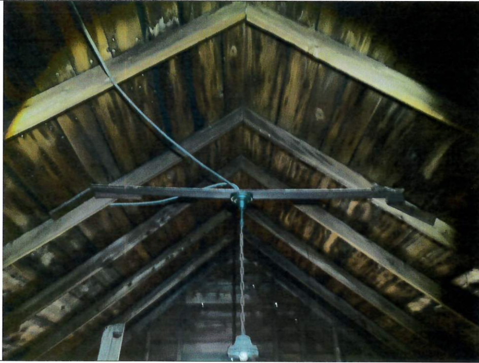
Photograph 9 – View of ridge and rafters looking west. Note staining at rafters and underside of roof boards.
