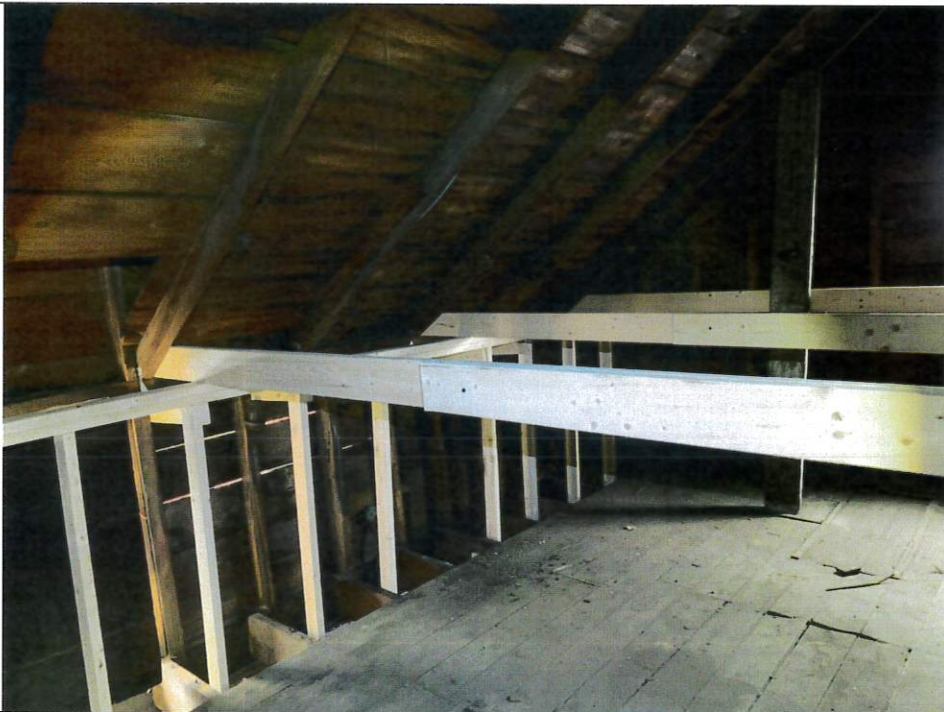
Photograph 10 – View of temporary rafter ties and shoring
