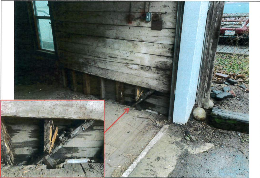
Photograph 5 – View of interior of east exterior wall. Note water seeping through boards and deterioration of studs and bracing.
