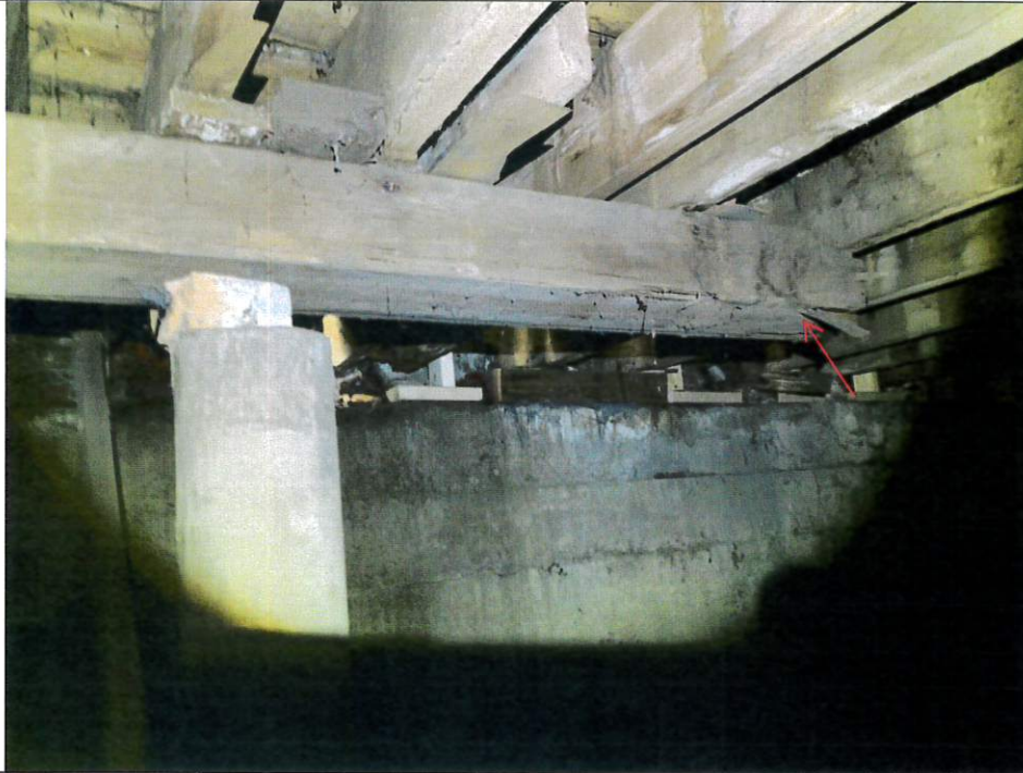
Photograph 15 – View of 4 \frac{3}{4} " x 8" girder near garage door opening. Note staining and collapsed west end of girder
