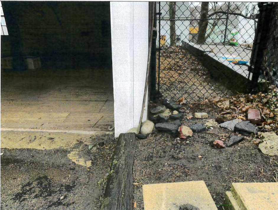
Photograph 4 – View of southeast corner. Note exterior grade is higher than the first floor elevation
