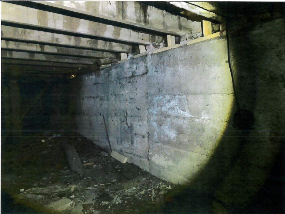
Photograph 18 – View cast-in-place concrete foundation wall at south (front) elevation
