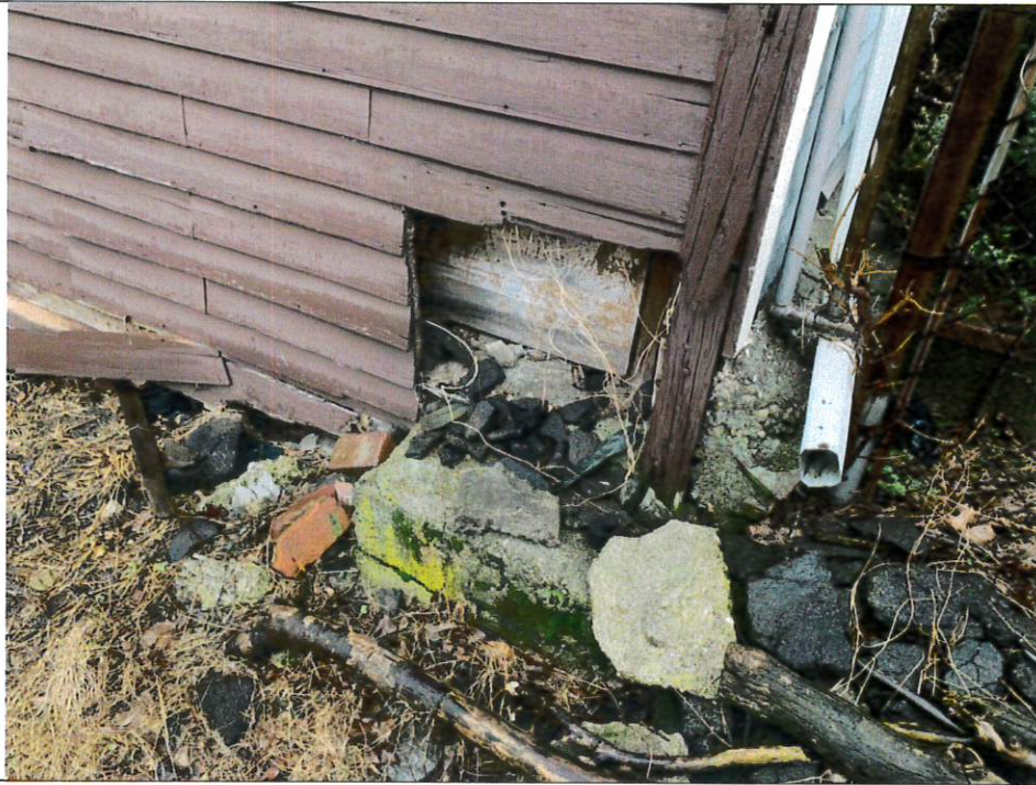
Photograph 7 – Closeup view of southwest corner, note deterioration at the top of foundation wall.
